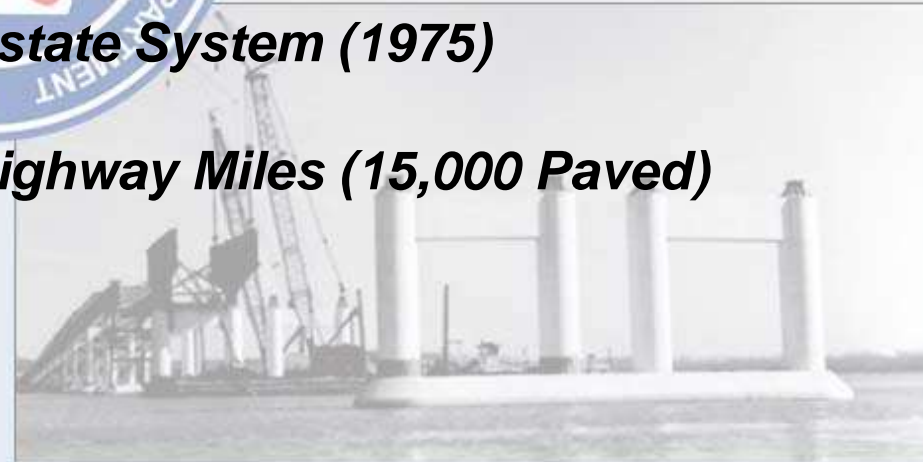
I-430 River Bridge, 1973
